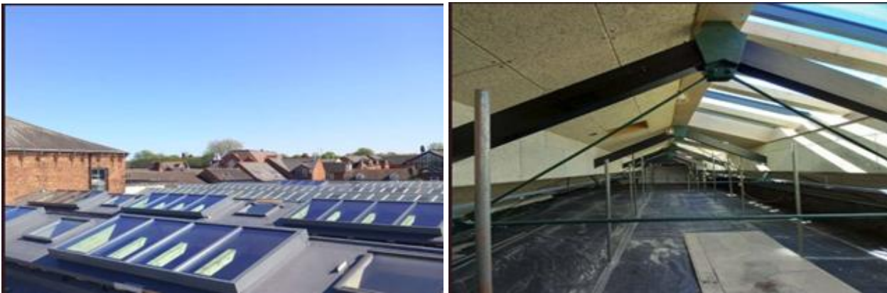
Pictures showing completed external roof coverings with new roof lights and internal eco-friendly Hereklith wood/wool insulation material.
